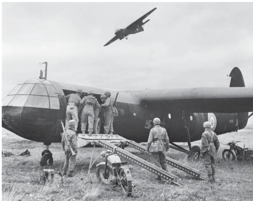
During an exercise at RAF Netheravon in December 1942, British airlanding troops unload Matchless 3G/L motorcycles, the standard British service machine, from a Horsa; they were intended for use by scouts and couriers. The Horsa's cargo door is lowered to serve as a loading ramp, but it was too fragile for the heavier loads. (IWM H 26215)
